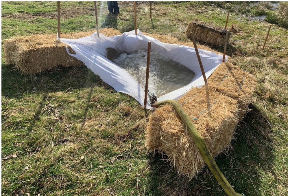
Figure 4: Standard Installation of Geofabric Filter Dam
